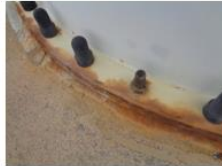
Figure 12 Tower bottom corrosion
