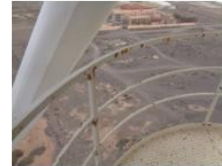
Figure 18 Corrosion at upper platform safety railing
