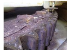
Figure 20 Corrosion at yaw gear and bolts
