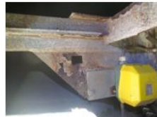
Figure 17 Corrosion at nacelle mainframe
