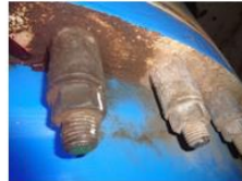
Figure 16 Corrosion at nacelle bolts
