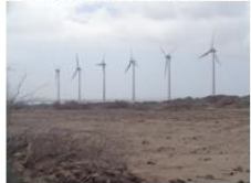
Figure 9 General view of 6 of the 11 wind turbines
