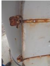
Figure 13 Corrosion at yaw gear and bolts
