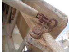
Figure 15 Corrosion at access ladder to nacelle
