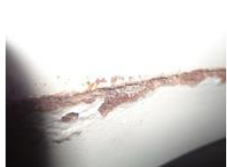
Figure 11 Tower mid joint corrosion - internal
