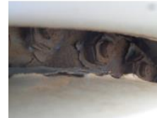
Figure 19 Corrosion at yaw gear and bolts
