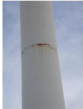
Figure 10 Tower mid joint corrosion - external
