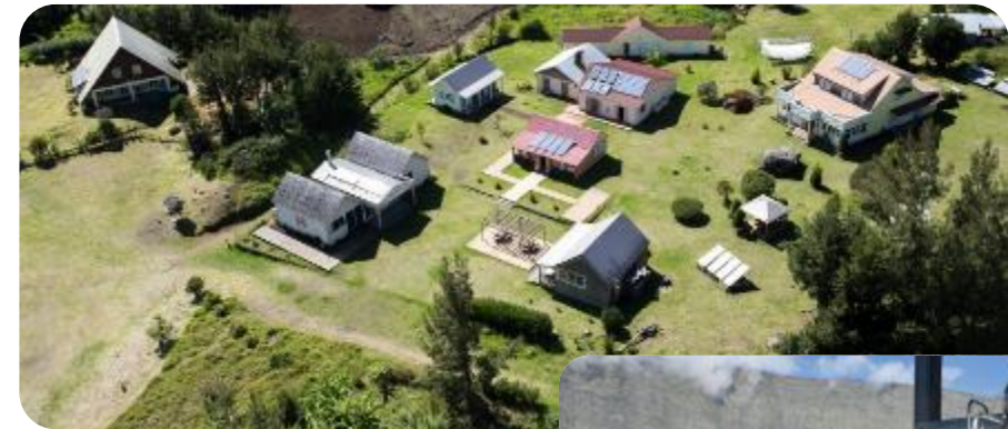
La Nouvelle – isolated site of Reunion Island Powidian facility in partnership with EDF SEI
